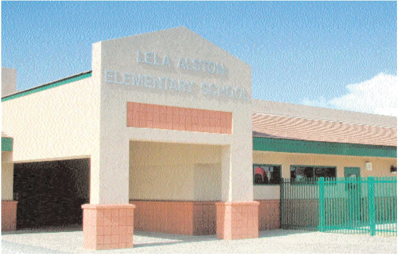
Lela Alston Elementary School in Phoenix, Arizona is a 40,500 square foot K-5 elementary school, with room for over 400 students. The school was built in seven months using modular construction.
